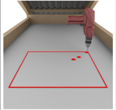
Drill a marker hole in ceiling to indicate one corner of the ceiling frame. Place two more holes to indicate direction of skylight.
