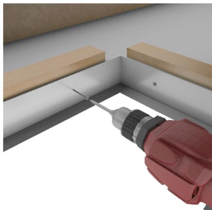
Secure the ceiling frame to ceiling by driving screws through ceiling frame collar into joists/trusses if available.
