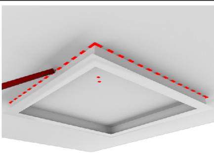
Back inside, using the direction holes as reference, place the inner ceiling frame corner against the corner hole.
