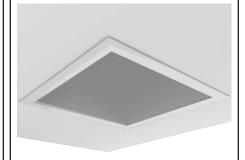
Let the diffuser panel rest flat inside the ceiling frame.
