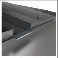
Rest the folded flat tabs of the aluminium shroud on the upstand on the soaker tray, so the flexi shaft hangs below.
