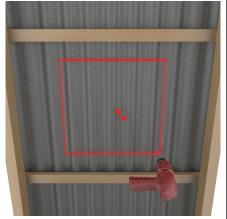
When satisfied with location, drill a hole in a bottom corner of throat position. Drill two holes above it to indicate direction of skylight.
