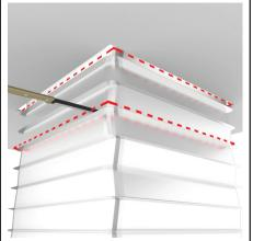
Using sharp knife and pliers/tinsnips, cut off excess flexi shaft t ribs below ceiling level.
