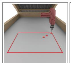
Drill a marker hole in ceiling to indicate one corner of the ceiling frame. Place two more holes to indicate direction of skylight.
