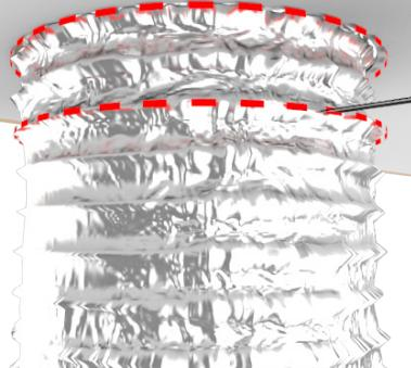
Cut off excess flexi duct 2 ribs below ceiling level.
