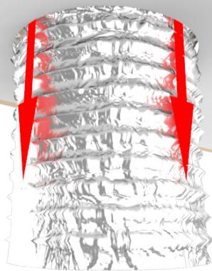
Pull excess flexi shaft through hole in ceiling.
