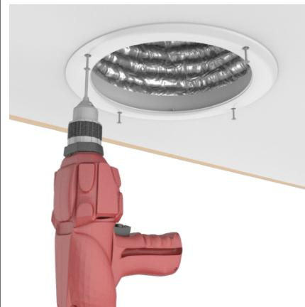
Using cordless drill, fix ceiling ring to ceiling with screws provided.
