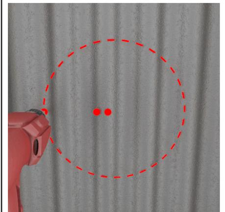
Using a drill, mark the edge of where the dome will be located on the roof sheeting.
