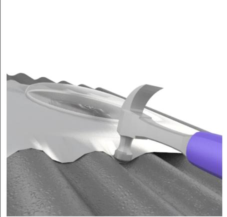
Using a hammer or rubber mallet, gently form the edges of the tray to match the roof profile.
