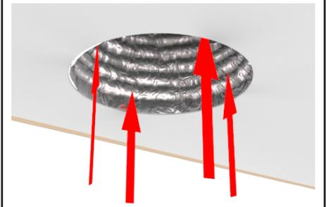
Push hanging flexi shaft back up into roof cavity.
