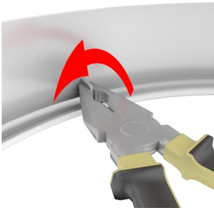
For non ventilated skylights: Using pliers, grip and twist white molded tabs inside ceiling ring to snap off.
