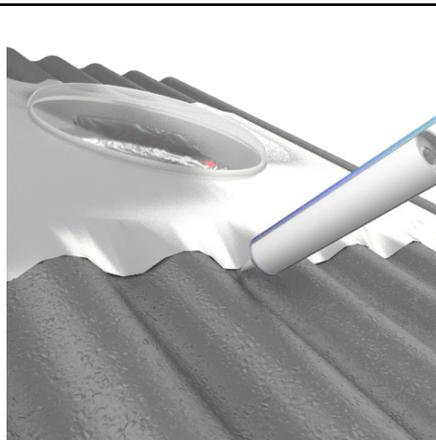
Use silicone to seal under edges of the top and bottom of the tray to roof sheeting.
